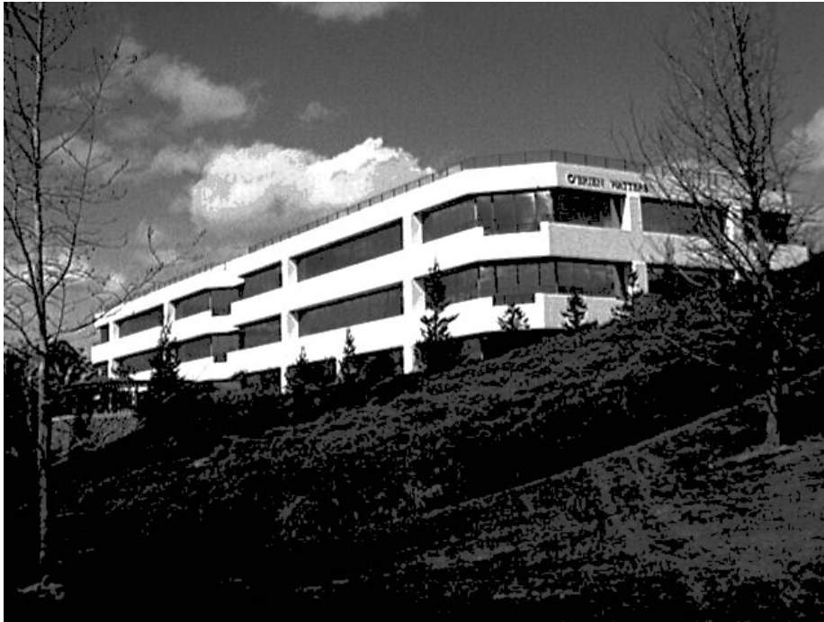
Fountain Grove Corporate Center One is one of Santa Rosa's premiere office properties and now features state-of-the-art energy efficient lighting.
